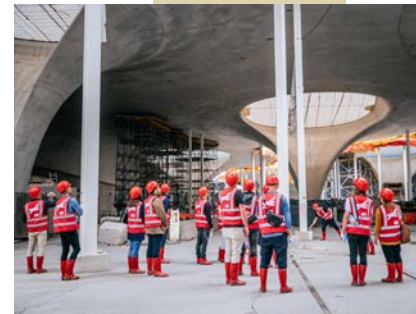
Fotos: Baustelle ITS © Thomas Niedermüller
